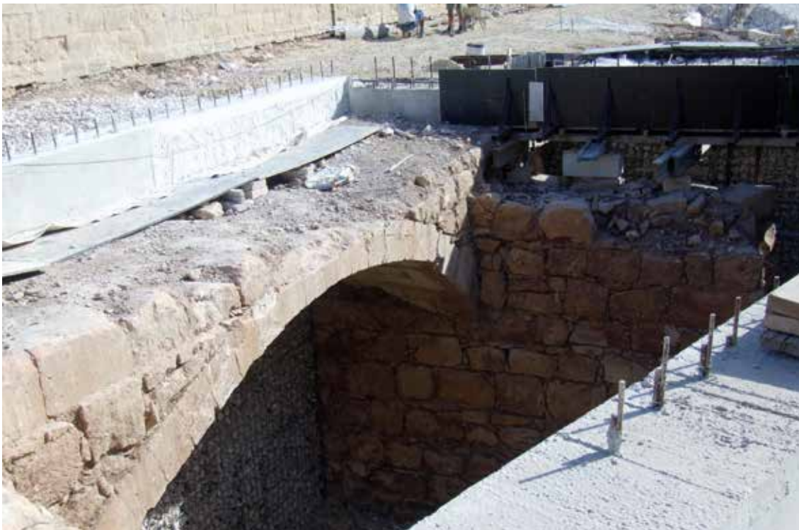
One of the 10 casemates discovered during the preparation works for the rehabilitation of Peacock Gardens in Valletta. The casemate was consolidated and was prepared as part of the interpretation of the garden. Image: Heritage Enterprise 2012.
